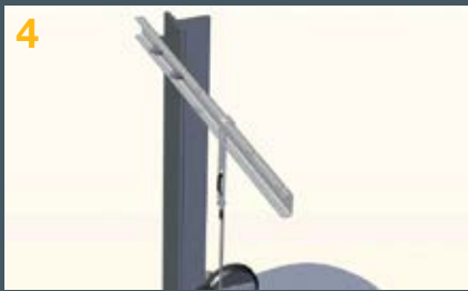
4 Standing on the car roof, the magnetic tape is rolled out during the ride down and inserted at the lower end in the tape suspension.
